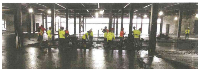
Fig. 2: A concrete placement on an elevated floor in a hospital in Ridgewood, NJ, USA. The concrete slab on a metal deck was reinforced using only synthetic macro fiber reinforcement
