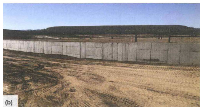
Fig. 5: Examples of projects constructed using FRC: (a) the slab-on-ground floors in this food processing facility in Troy, OH, USA, were designed and constructed using FRC reinforced with steel fibers only; and (b) the retaining walls for a flood control project in Tucson, AZ, USA, were constructed with synthetic macro fibers designed to replace 40% of the steel bar reinforcement determined during preliminary design
