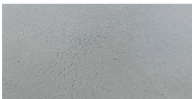
Fig. 3: Surface cracking during troweling operation, concrete below surface is still plastic
