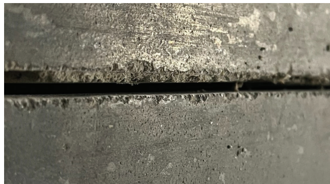
Fig. 9: Saw cutting too early results in raveled joint edges (photo courtesy of Scott Metzger, Metzger/McGuire)
