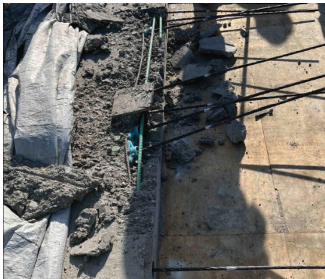
Fig. 12: Tendons in a concrete slab constructed with Type II concrete were stressed based on a maturity calibration for Type I cement concrete. The strength of the Type II cement concrete was overestimated, resulting in slab blowouts
